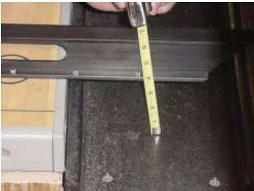
*Determining the Shallowest Part of Gutter with a tape measure and level*
